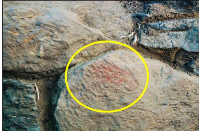
Photo 12. Close-up of plaster location on west wall of foundation. Note the reddish color, possibly paint.
