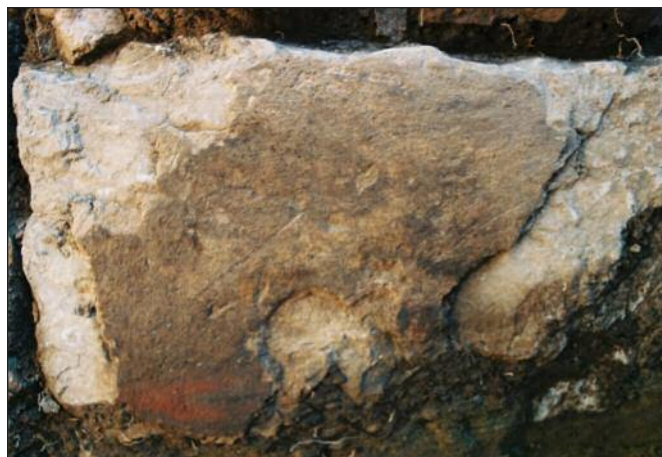
Photo 7. Close-up of the one plaster location on inside east wall of foundation.
