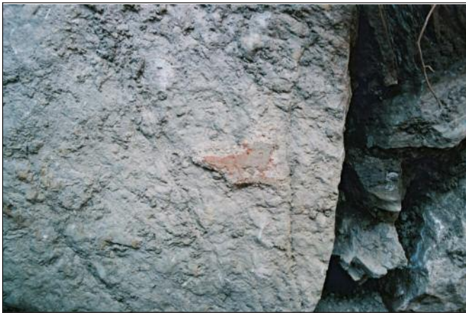
Photo 14. Close-up of upper left plaster location on north wall of foundation. Note reddish color.
