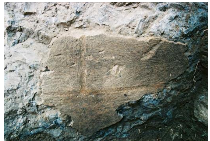
Photo 16. Close-up of lower right plaster location on north wall of foundation. Note the rectangular pattern of incised lines on the surface.
