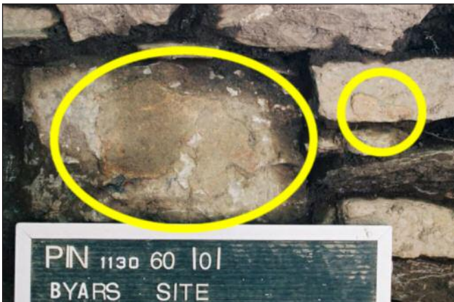
Photo 9. Close-up of two of the three plaster locations on the south wall.
