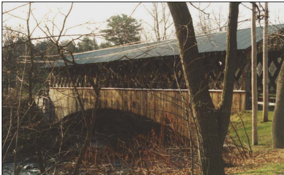
Photograph 2. Looking Southeast Toward the Wooden Pedestrian Bridge Located near the Southern Boundary of the Vroman I Site. This bridge is located outside the current project limits and will not be impacted during the realignment of the Route 443 and Route 30 intersection.
