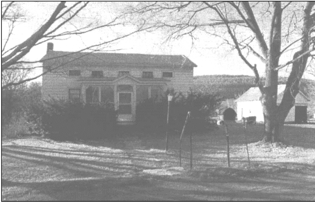
Photograph 3. Looking West Toward the Former Dietz Residence (MDS 1). This building was removed in 1997 and only remnants of the foundation remain within the project limits. As shown in this photograph, several buildings formerly stood near the residence that were associated with the occupation of the property during the mid-/late nineteenth and early twentieth centuries.
