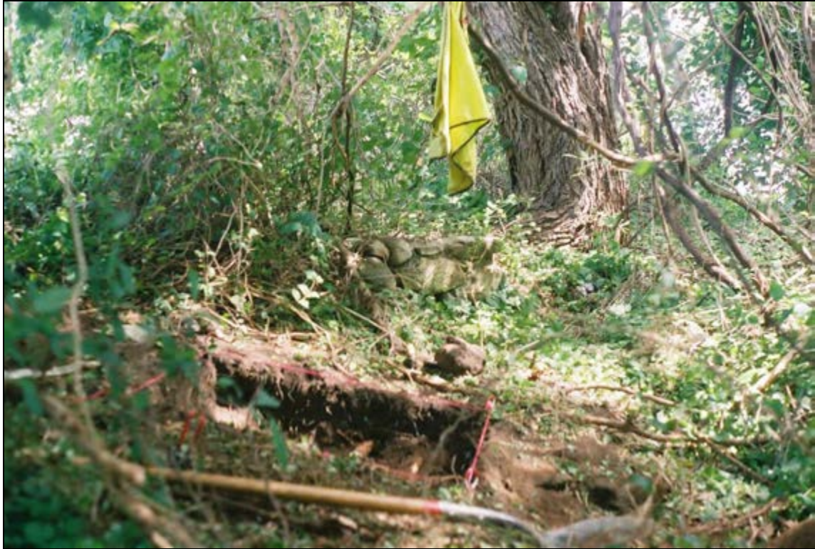
Photograph 26. The Extant Wall (just below the hanging safety vest), Looking North
