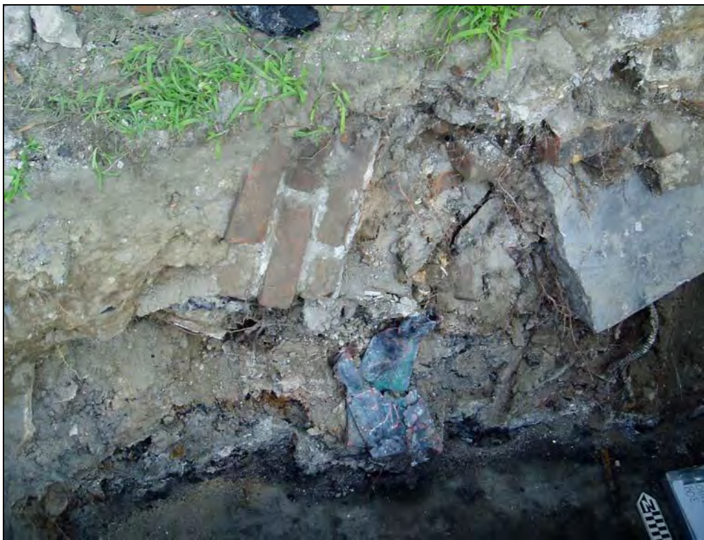
Photograph 45. Architectural Debris in the North Wall of Unit 47
