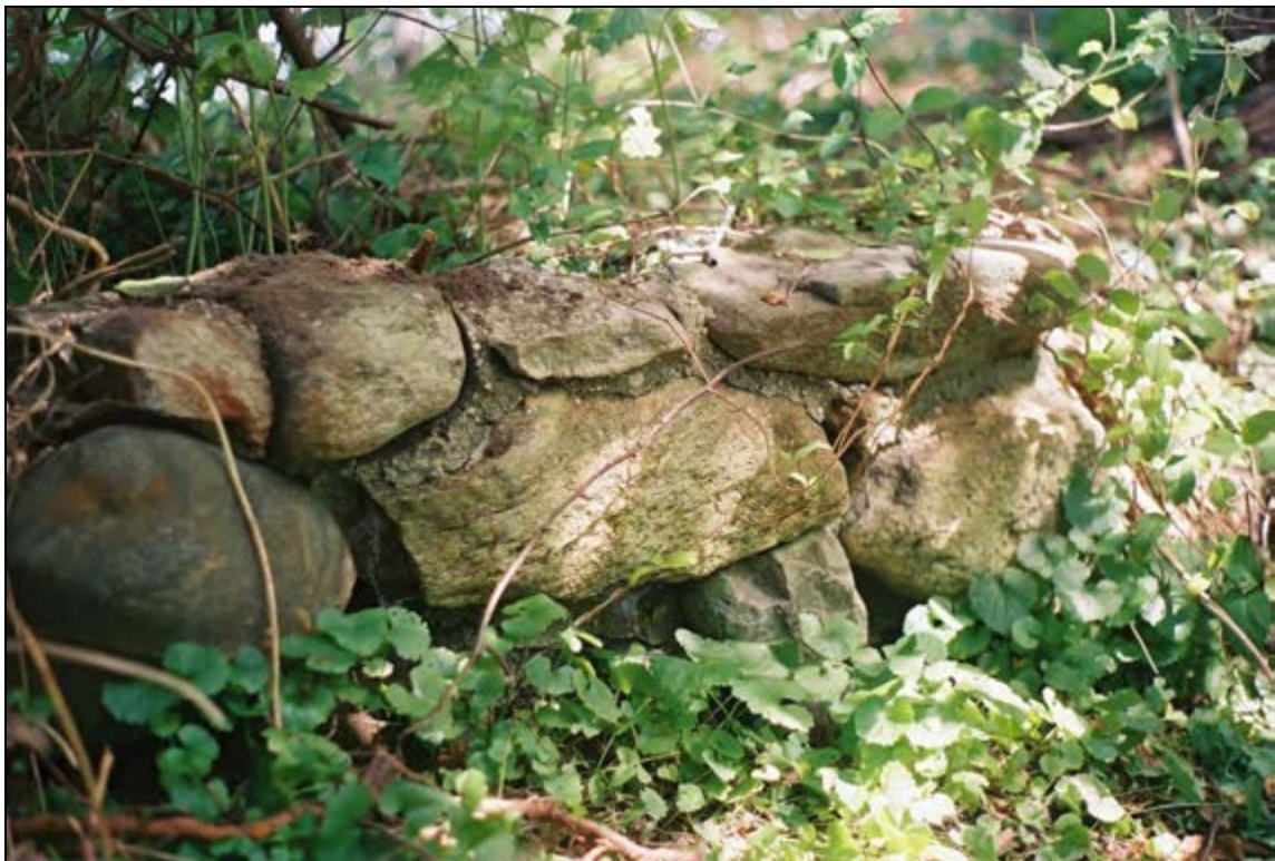
Photograph 27. Close-up of the Extant Wall, Looking North
