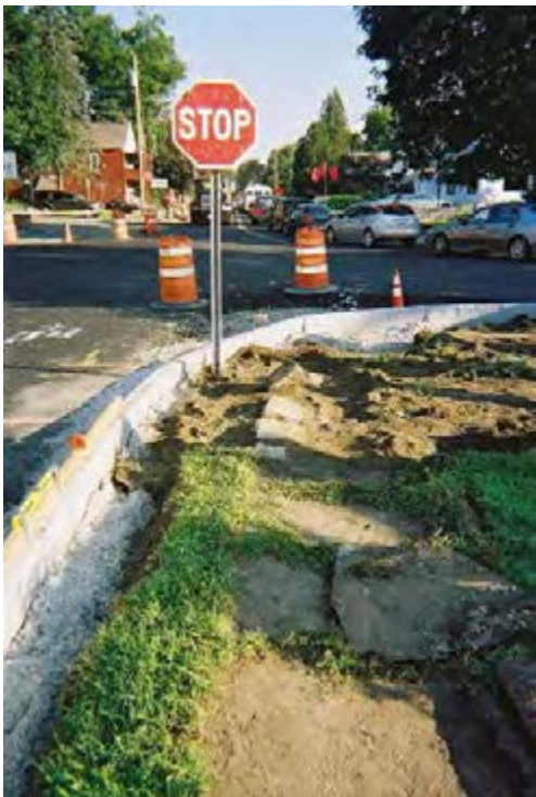
Photo 7.28: View north of the stone retaining wall at the corner of Montgomery Street and Broadway after the removal of the sidewalk slabs that concealed it.
