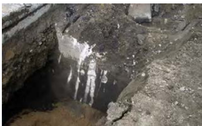
Photo 10.13: View northwest of the poured concrete abutment in Incident 177. Note the impressions of the wood forms on the south face of the wall.
