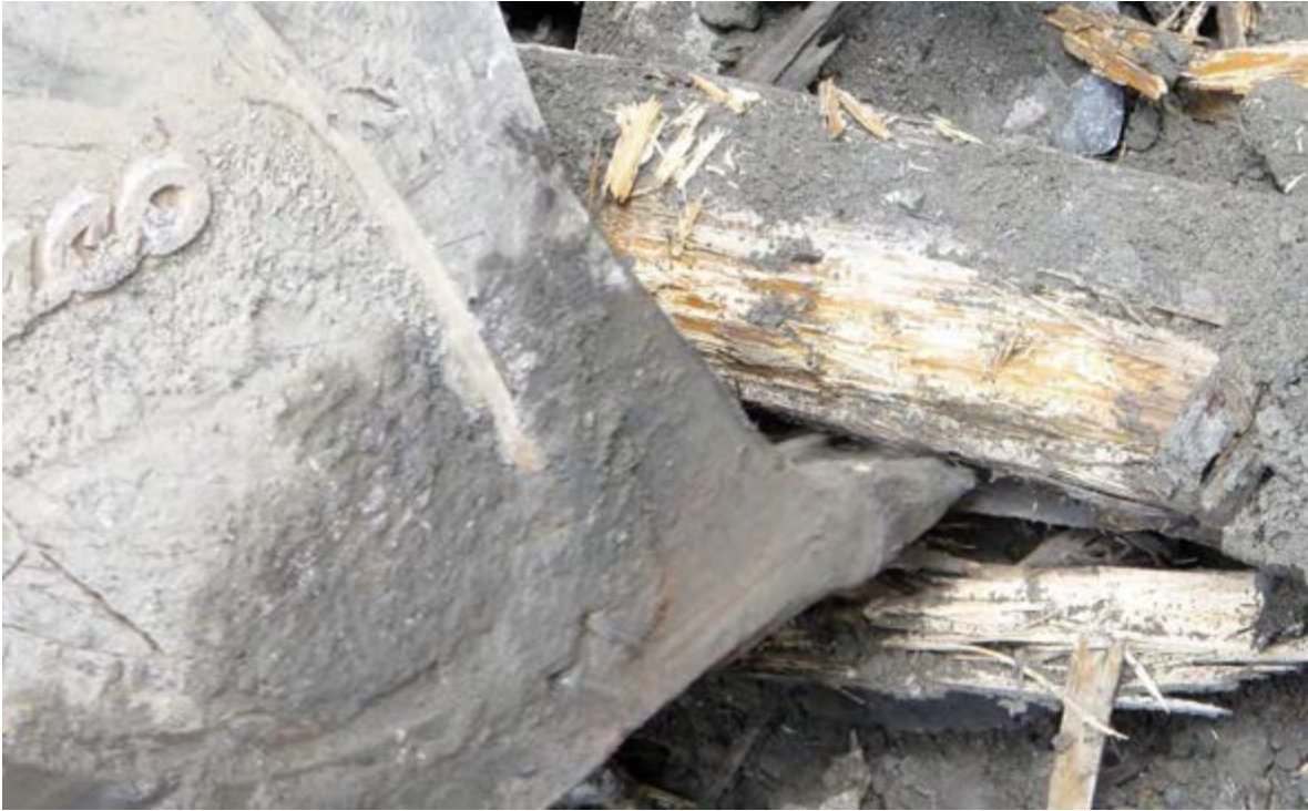
Photo 10.10: Wood timber at the bottom of the trench during removal by the backhoe bucket.
