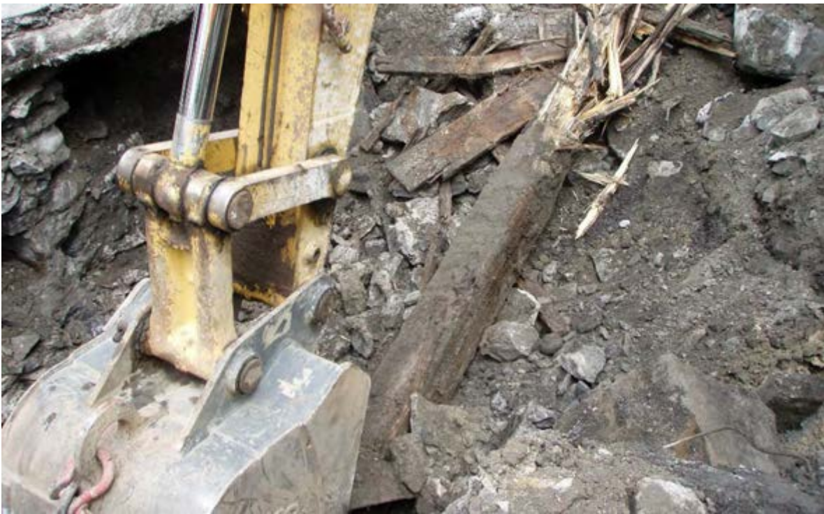
Photo 10.11: Wood timber and flat planks removed from beneath the dismantled stone feature.
