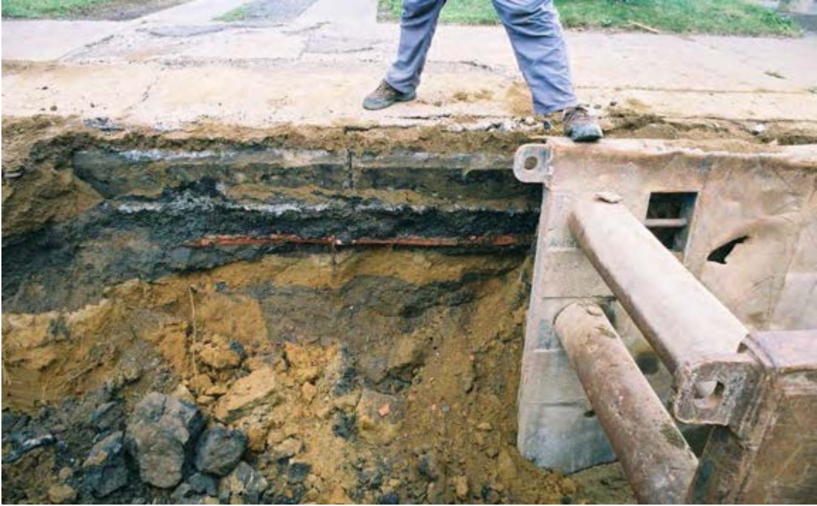
Photo 12.6: View west of the redware drainage pipe in situ , beneath the west curb in front of the house at #85 Broadway during new waterline construction.
