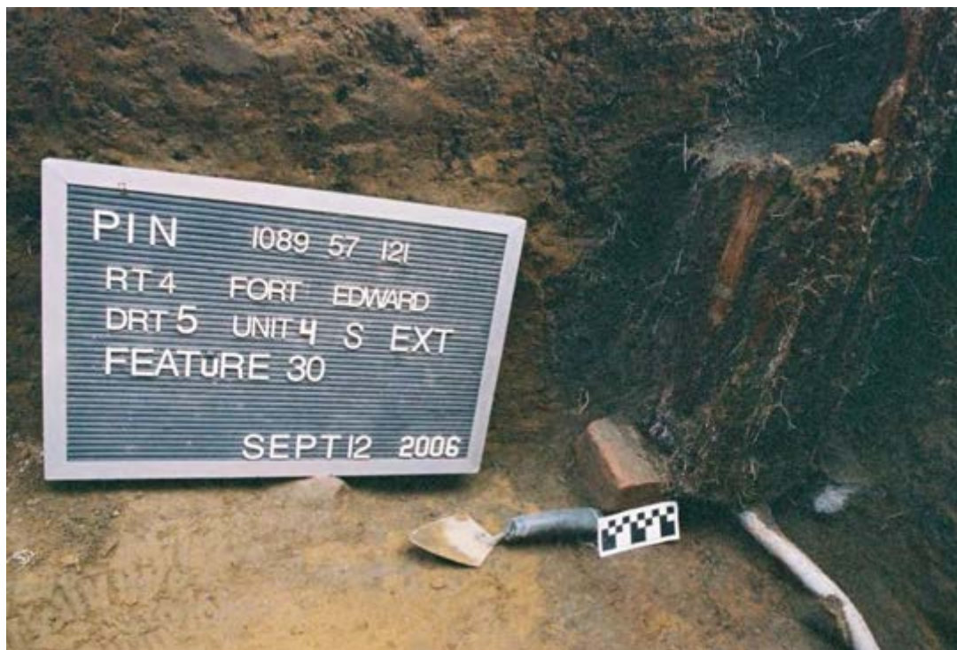
Photo 7.13: View of the base of the wooden valve box where it rested on a brick and a rock just above the shut-off valve to the lead pipe.
