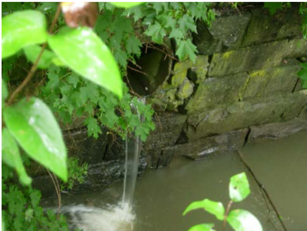
Photo 7.23: Interior of the culvert in 2013 showing the 19 inch storm sewer emptying into the creek from the bed of the Old Champlain Canal below the former aqueduct.
