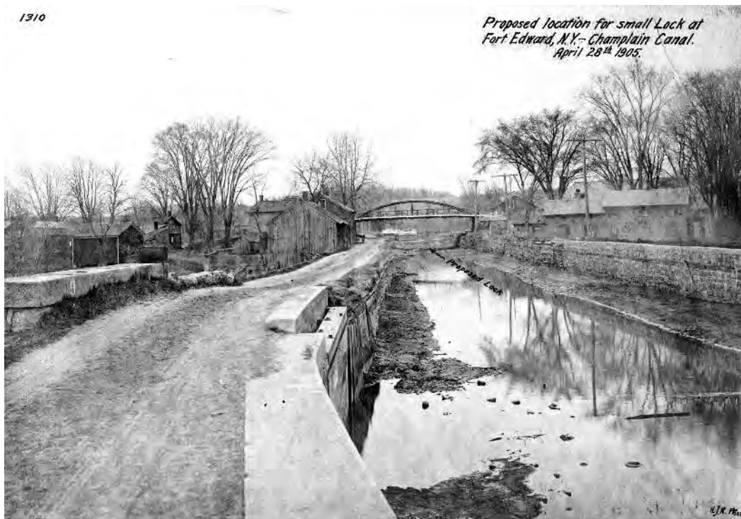
Photo 7.20: The aqueduct in 1905 with the water drained, looking south towards the Argyle Street bridge showing the future site of the Junction Lock. The capstones of the aqueduct arch are visible at far left (NYSACD).
