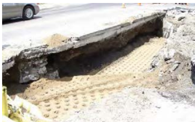
Photo 10.14: View northwest of the drain line construction trench between Feature 1 and Feature 2, the south and north bridge abutments in Incident 177. The new pipe was buried and covered with clean sand, but the cinder fill is still visible along the west trench wall.
