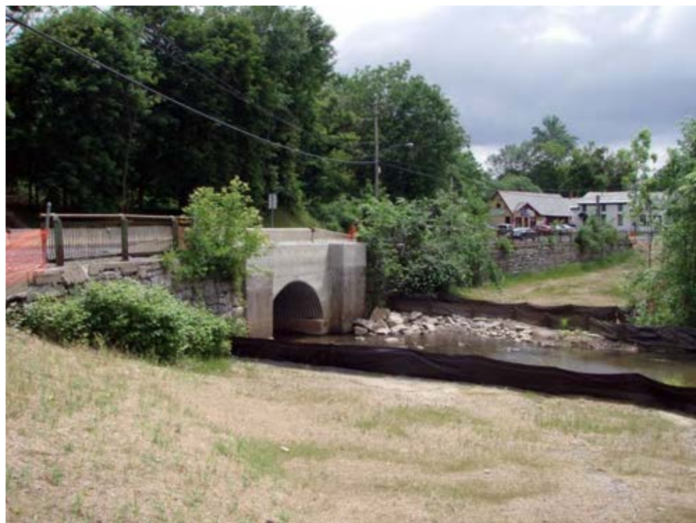
Photo 7.17: The viaduct in 2007, looking south. This view shows the walls built in 1869 with today's new concrete reinforcement lined with corrugated steel enclosing the box culvert inserted in 1968.
