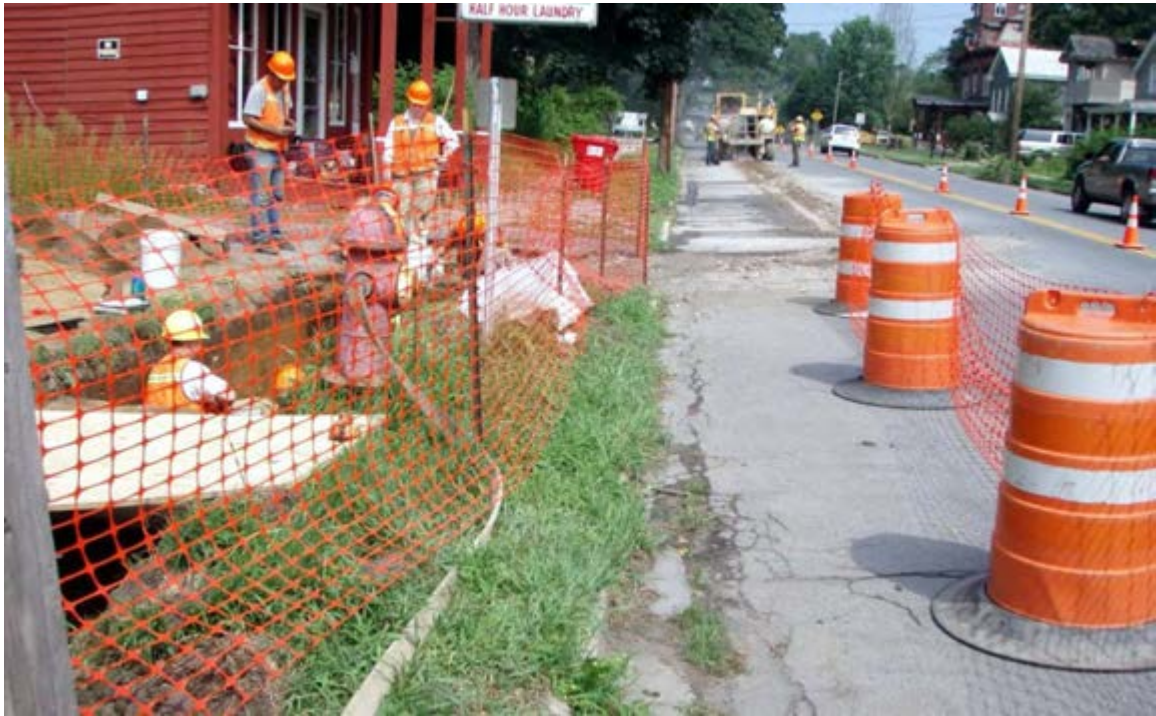
Photo 1.1: View north of unit excavations underway in sidewalk alignment of DRT 1 while pavement saw cutting is occurring in the street to the north in preparation for pavement removal in the remainder of DRT 1 as well as for DRTs 2 and 3.
