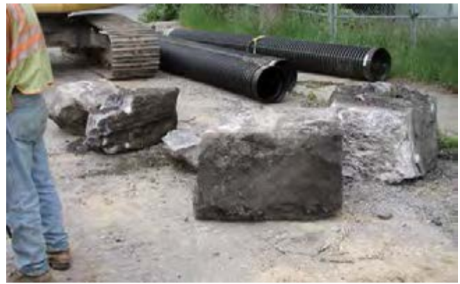
Photo 10.9: Some of the large cut stones removed from the abutment in the drainage trench in Incident 177.
