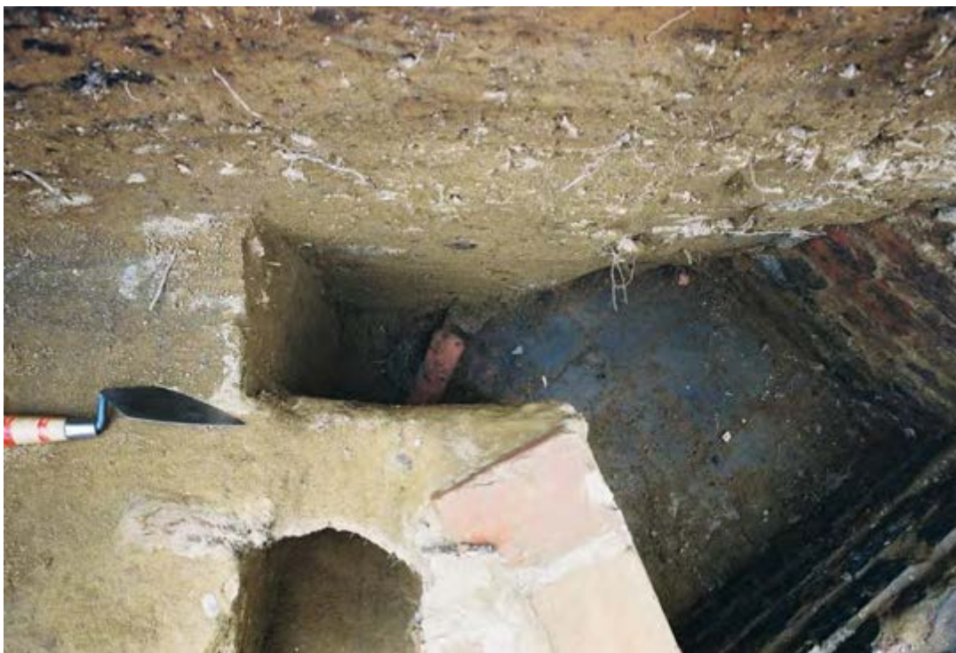
Photo 6.17: View from above showing the wood timber, the nail, and the bricks facing the curved hearth front.
