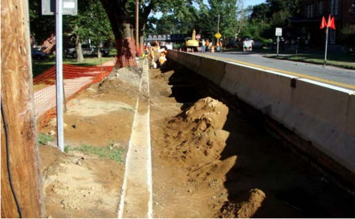
Photo 1.4: View north of DRT 2 nearing completion of unit excavation. As units were completed, some were used as spoils containers for screening soil.
