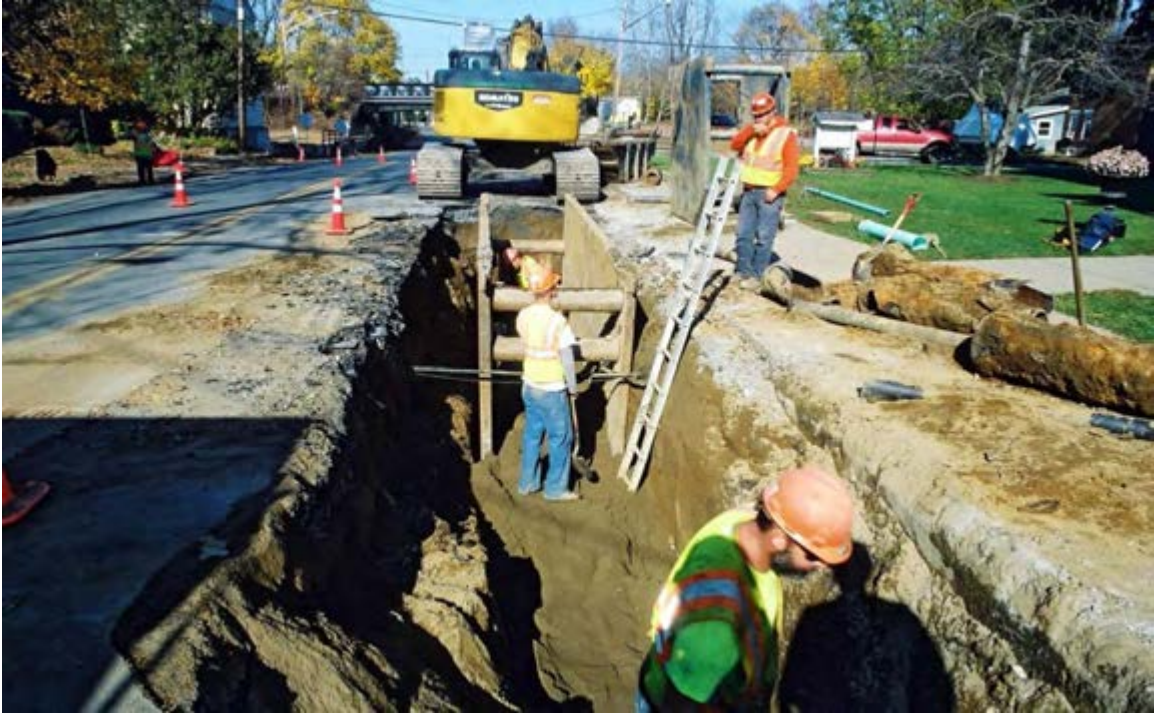
Photo 1.6: View north of partially backfilled section of trench (foreground) while new sewer pipe is being installed within trench box in background (Incident 100).
