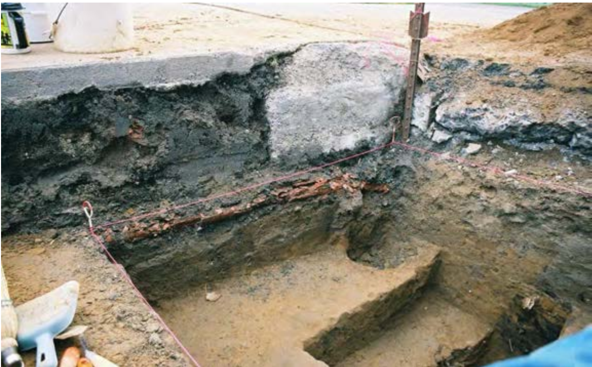
Photo 12.7: View southeast of the redware drainage pipe under the east curb in front of #82 Broadway (Unit 1 in DRT 5) prior to new sewer line construction.
