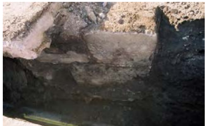
Photo 10.6: View west of the mortared cut stone structure (probable canal bridge abutment) in Incident 101 at SM 17+993. The black plastic gas line lies at the bottom of the trench.
