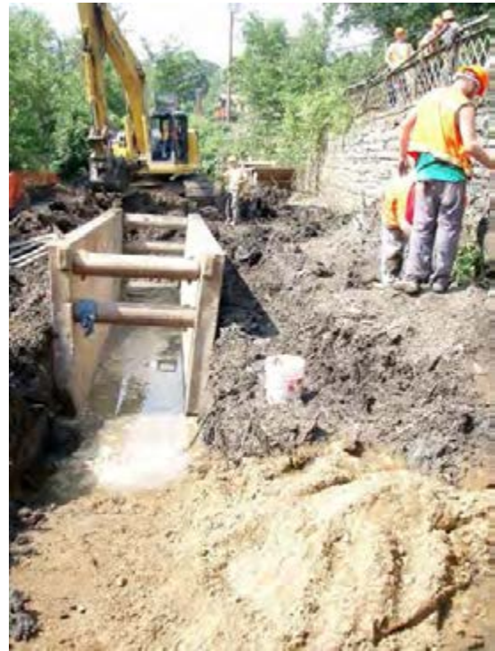
Photo 7.25: View north of waterline construction trenching along the base of the viaduct wall.
