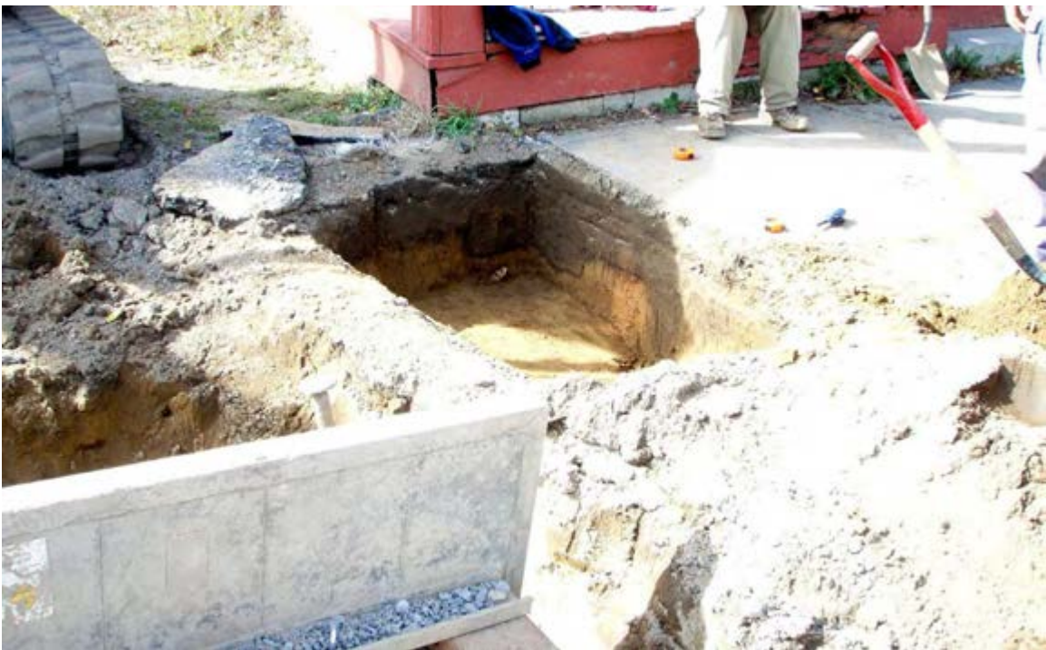
Photo 1.10: Unit excavated manually where a large slab of stone sidewalk was removed during trenching for water service connection to the structure (Incident 81).
