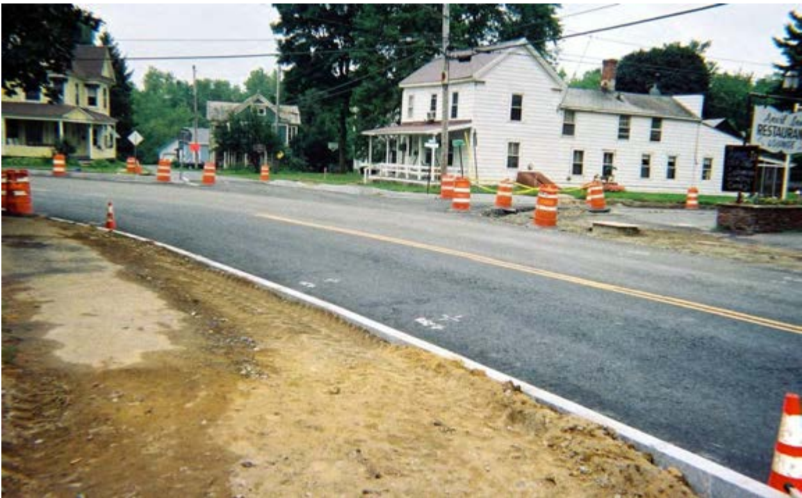
Photo 4.4: View south of the curve near Montgomery and Edward Streets during fall of 2007. The new utilities were complete, the old road surface and curbs had been removed, and new base layers and curbing installed. The Anvil Inn Restaurant is at right just out of the photo.
