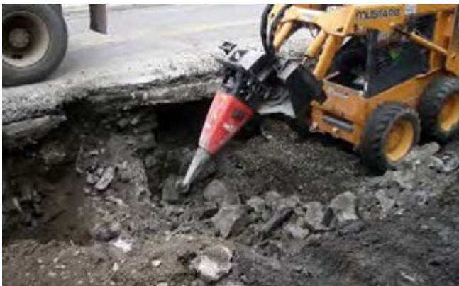
Photo 10.8: View northwest of the hoe ram battering apart the feature to progress the drainage line trench northward.
