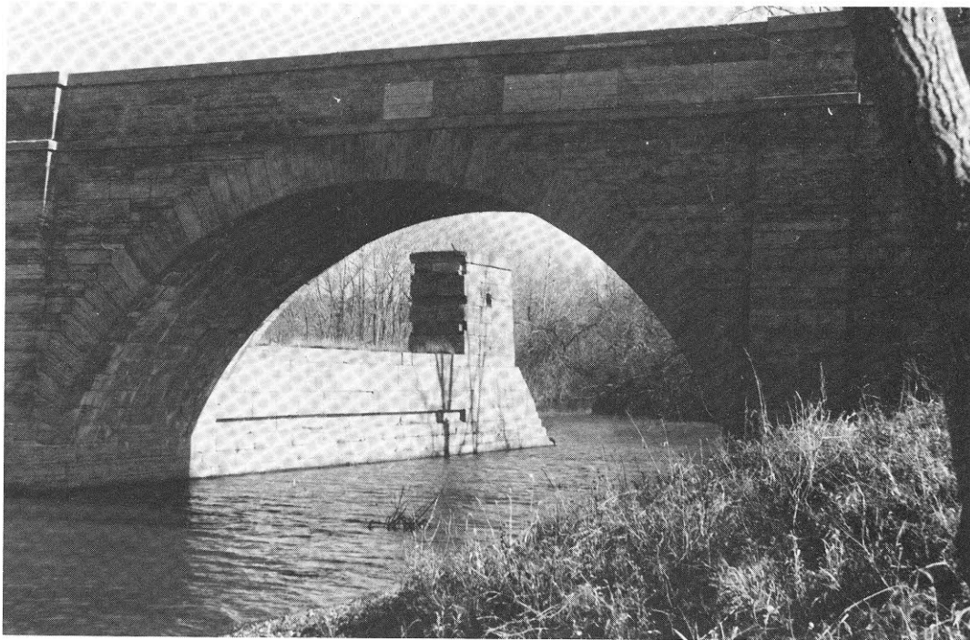
Figure 8. Close-up of vaulted archway of Erie Canal viaduct over Schoharie Creek.
