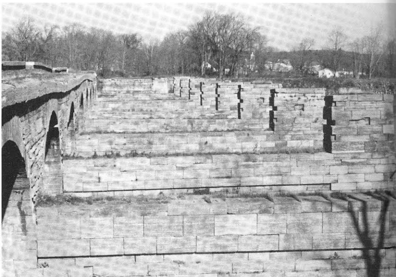
Figure 7. Viaduct for old Erie Canal over Schoharie Creek, looking east toward Fort Hunter; note towpath on left.
